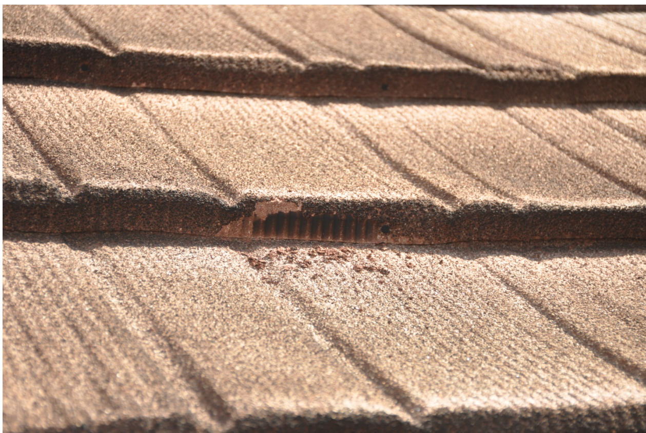
Figure 4.1.2: Close-up of decomposition of Natural Stone Coating
