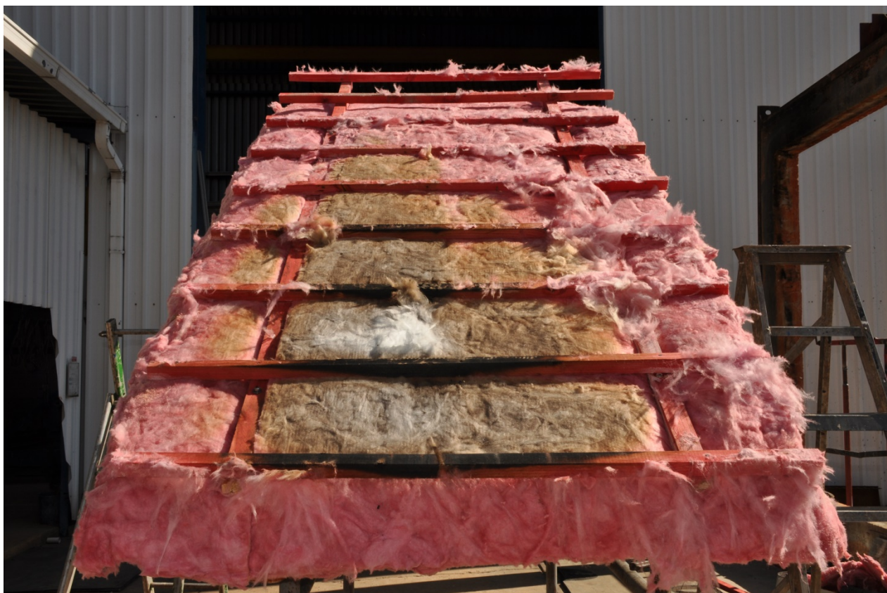
Figure 4.1.9: Bottom layer of Pink Aerolite under Pine Brandering and Bearers
