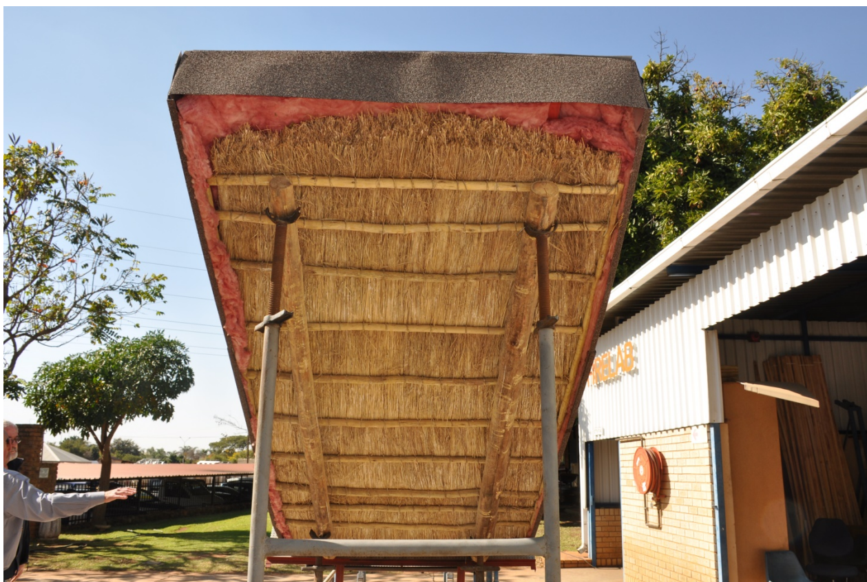
Figure 2.2: Harvey Thatch Tile System as seen from the unexposed (Interior/Room) side
