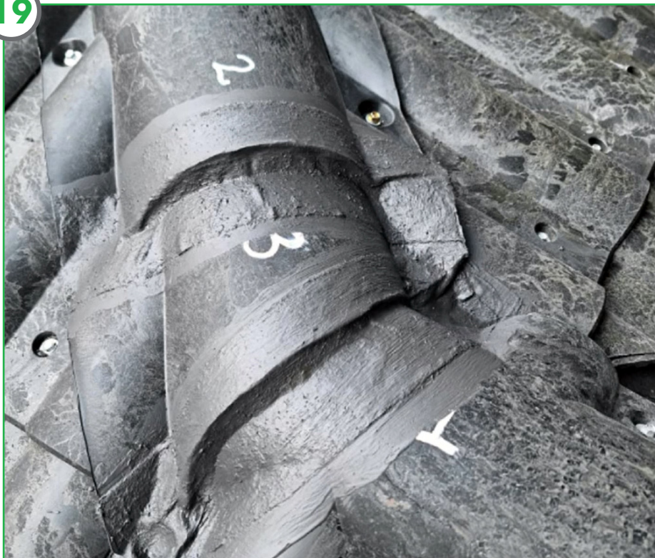
After sealing ridge cap gaps with FIBASTRIP® and LIKWID RUBBER®
